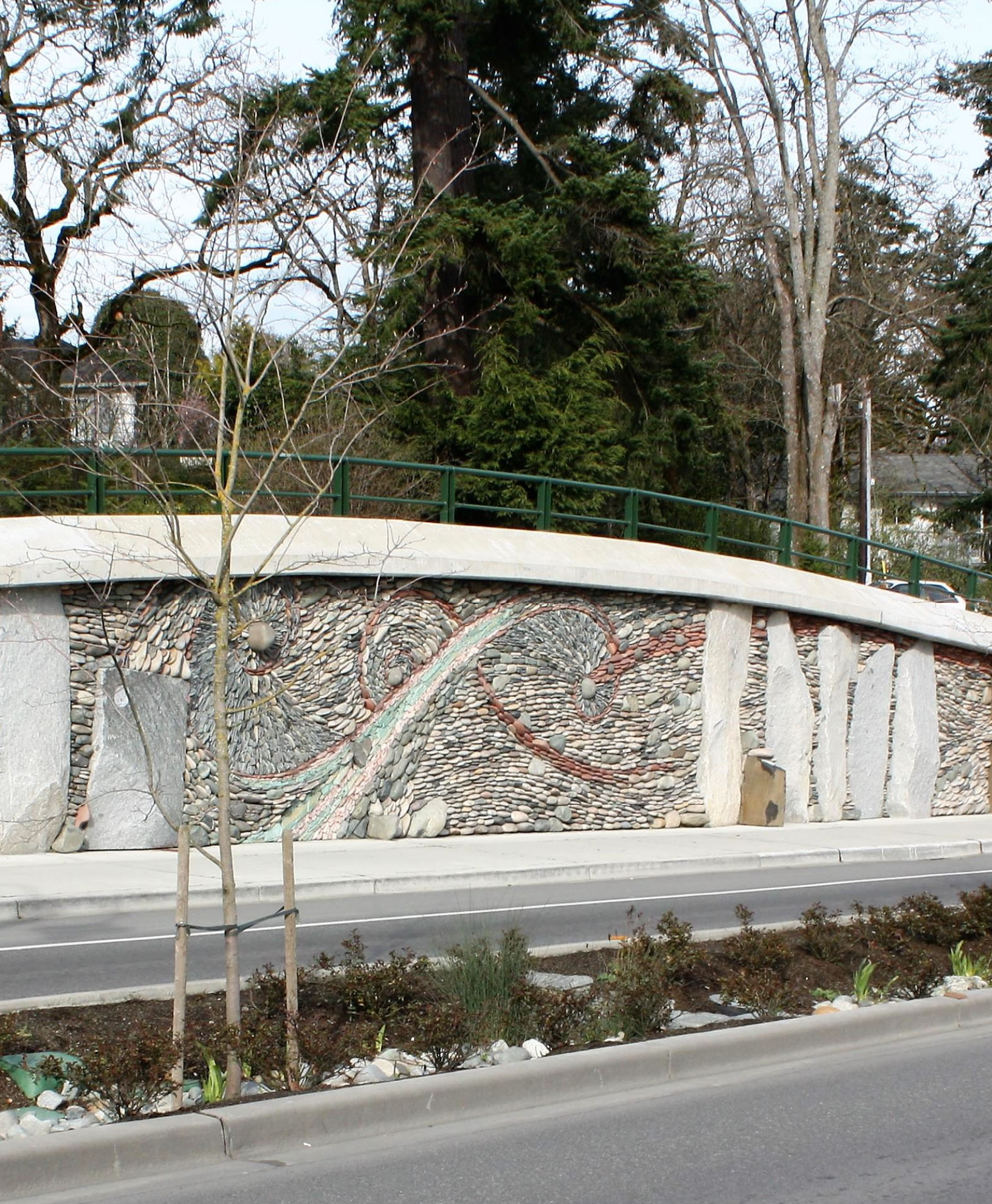
Stone wall on Island Highway
